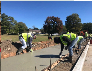
City of Atlanta workers build a new sidewalk in front of Sadie G. Mays.
