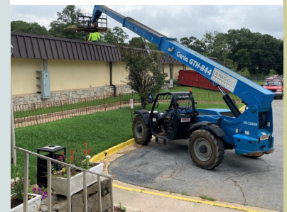
Atlanta Roofing truck deposits materials on the roof at SGM.
